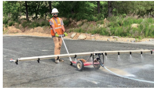
图11 微生物固化飞机跑道 [9] Fig.11 Microbial solidification of airstrips [9]
